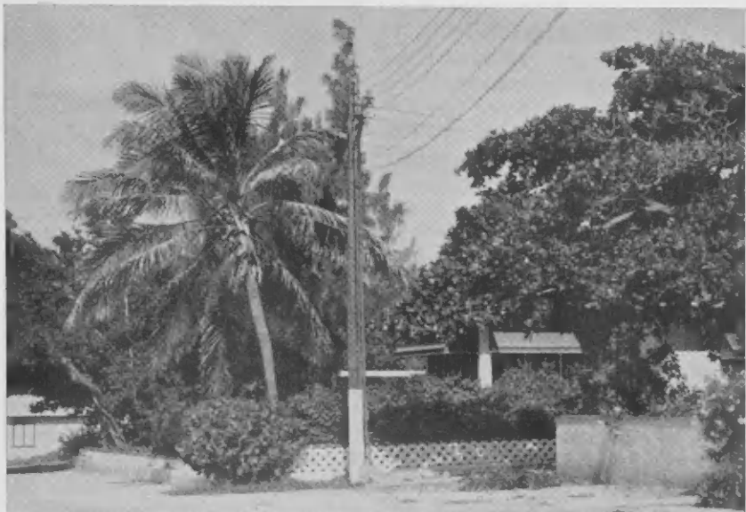
ELECTRIC WIRES passing through trees are dangerous. WAYA ELECTRICO cu ta pasa den palu ta peligroso.
